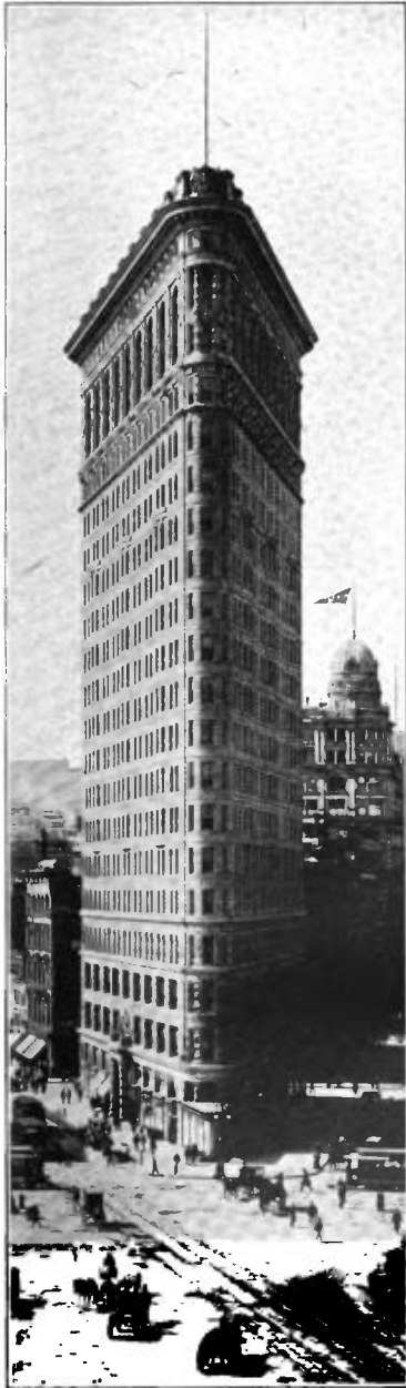
Copyright 1903 by Detroit Photographic Co. Fig. 131.—“Flat-Iron” Building, New York. (For method of construction, see STEEL CONSTRUCTION, and Plate II., Fig. 4, of that article.)
