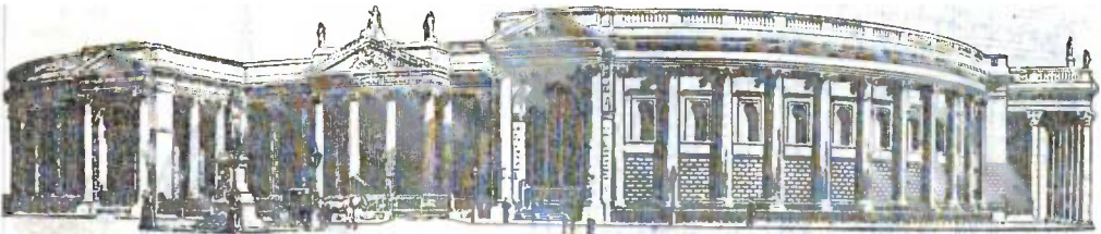
FIG. 85.—Bank of Ireland, Dublin.
