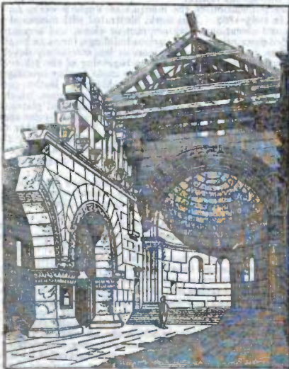
FIG. 32.—Interior of the Church of Kalb-Lauzeh.
